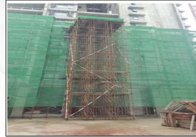
material loading platform
