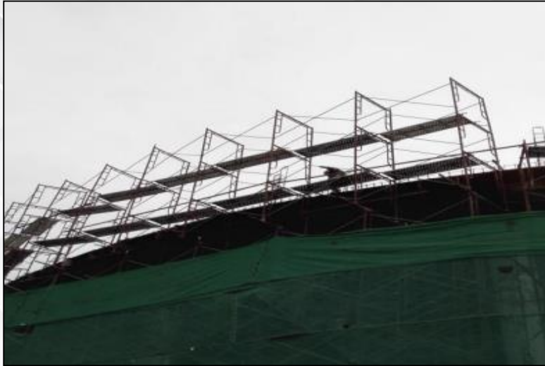
Provided platforms for every levels
