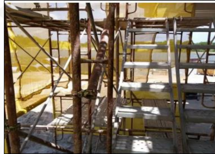
Scaffold access and egress
