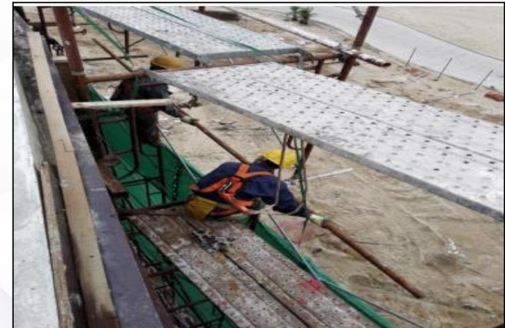
Installed horizontal bracing for scaffold
