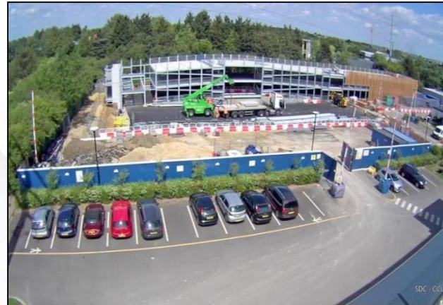
Car park area
