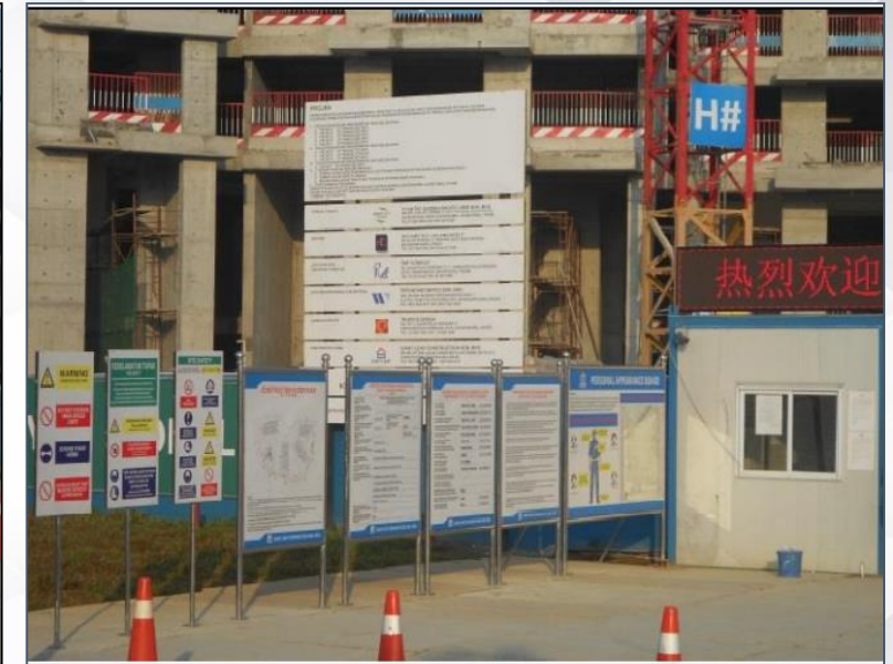
Notice board and safety sign at entrance
