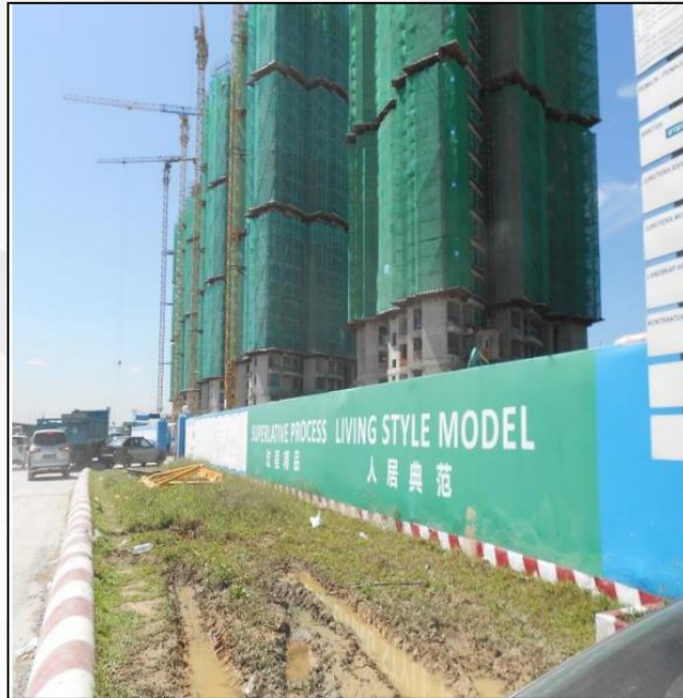
Assembled wall (fence)
