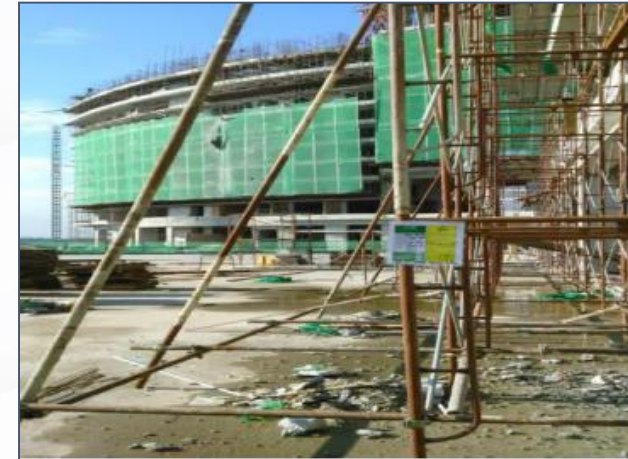
Additionally provided outrigger support
